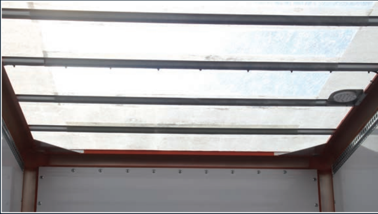
GRP translucent roof panel
